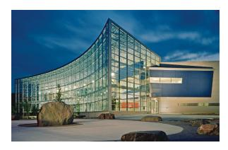
Oriented to promote natural lighting and take advantage of site elements, the Taubman Center's low-e glass skin is designed to reduce heat loss and maximize daylight without succumbing to excessive solar heat gain.
